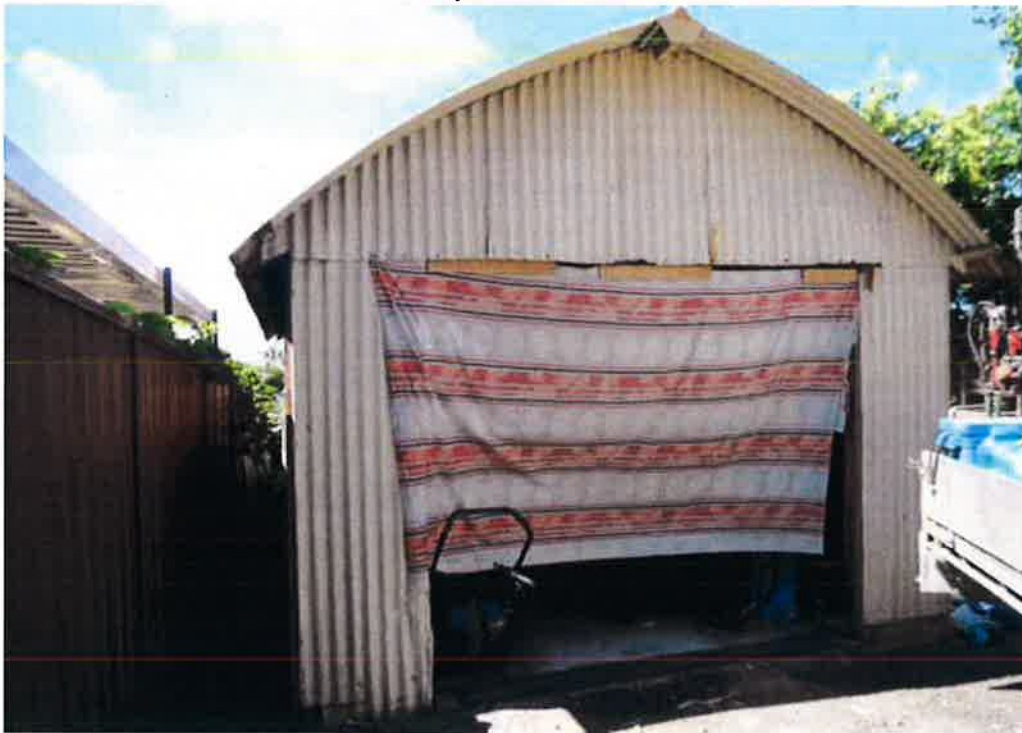
Photograph 14 Rear of 6 St Hilliers Rd, showing shed. Sample F1-A (asbestos cement) collected from left of shed
